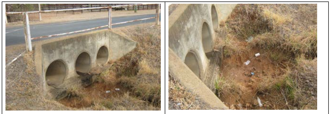
Figure 7-2: Existing Stormwater Outlet 1
