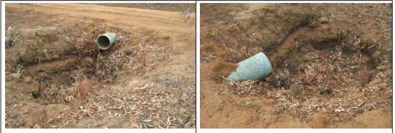
Figure 7-3: Existing Stormwater Outlet 2
